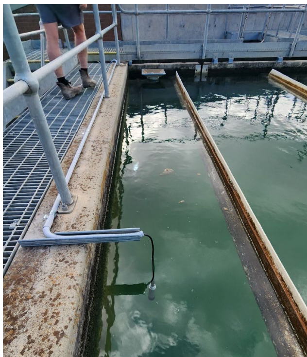
Hanging high range turbidity sensor
